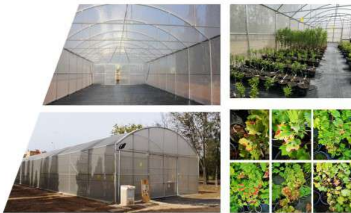
Figure C.2: Experimental setup. Greenhouse facilities and general view of its interior and the arrangement of the vine plants. The metallic structure is covered with an anti-thrips mesh.
