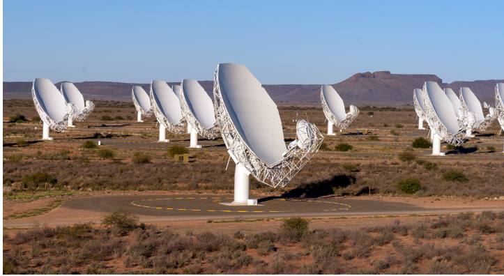
Figure 6.1: The MeerKAT radio-interferometric array in South Africa. It consists of 64 antennas, and will be a part of the future Square Kilometer Array (SKA).
