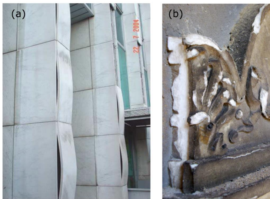
Fig. 8 Marble bowing and sugaring. (a) Bowing of marble slabs on Zagrepcanka business tower in Zagreb, Croatia (Grelk et al. 2007), and (b) sugaring on gravestones in the Monumental Cemetery in Bologna, Italy (Sassoni et al. 2014).
