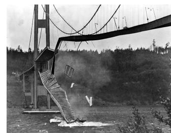
Figure 5.2: Tacoma Narrows bridge collapse, Nov. 1940.
