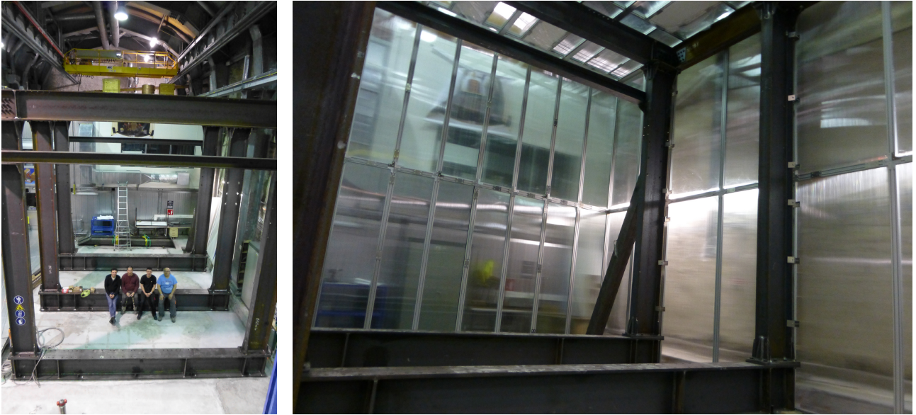
Figure 3.3: (left) Picture of the integration iron support structure at the location of the former NEMO-3 experiment at LSM. (right) Picture of the inside of the clean tent (before general cleaning) installed on the support structure with the top fanjets blowing clean air (right).
