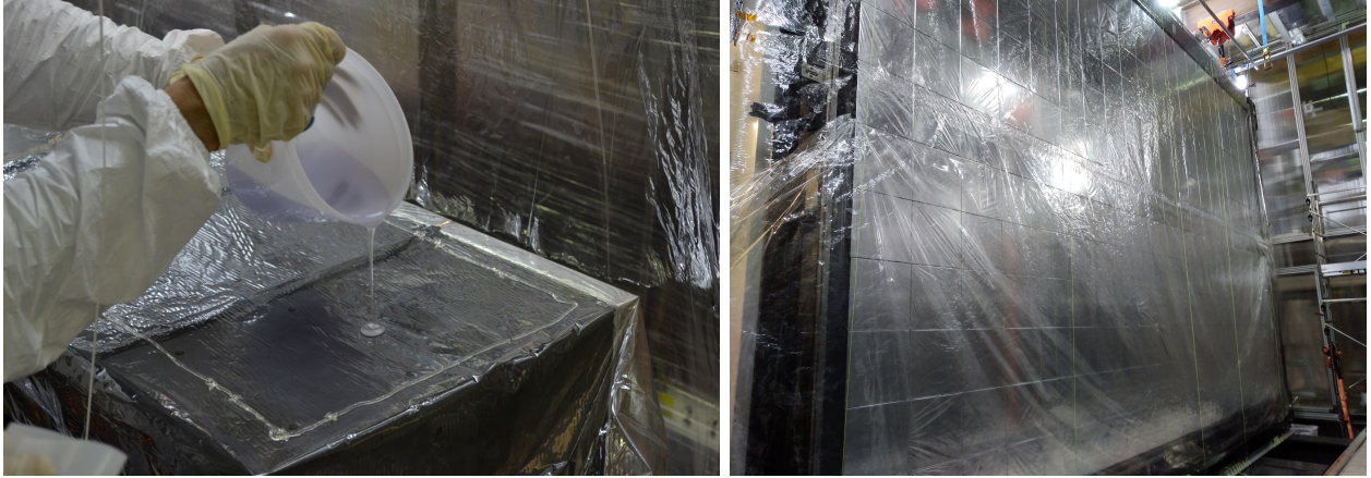
Figure 3.25: (left) Pouring of stycast glue on top on a nylon film after completion of a row of calorbrick of the first calorimeter main wall, before placing the next film already hanging in the back. (right) Gas tightness of the second calorimeter main wall ensured by the gluing of two nylon films together directly in front of the calorimeter wall, populated with all its calorbricks.
