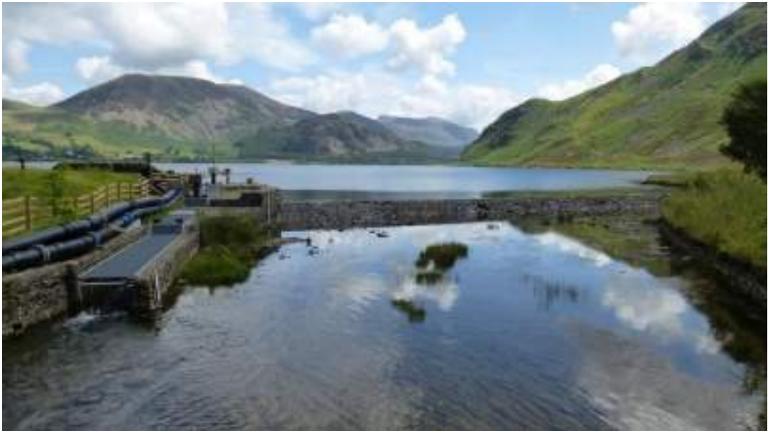
Plate 1.1. Outlet of Ennerdale Water, with the weir and fish-pass (left hand-side). When lake levels are low, the weir does not overflow and compensation flows are released through the fish-pass (Photo: Baptiste Marteau).
