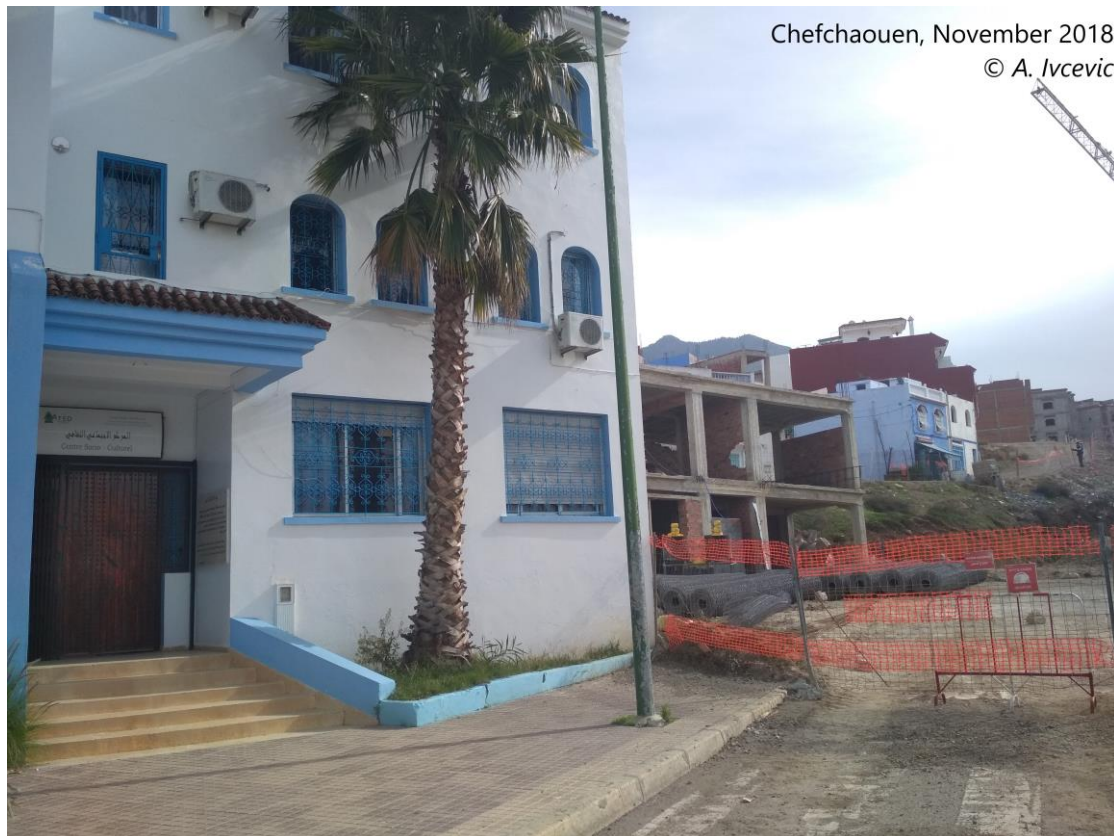
Figure 23: Landslide stabilisation works just in the neighbourhood of my interlocutor's association from Chefchaouen.
