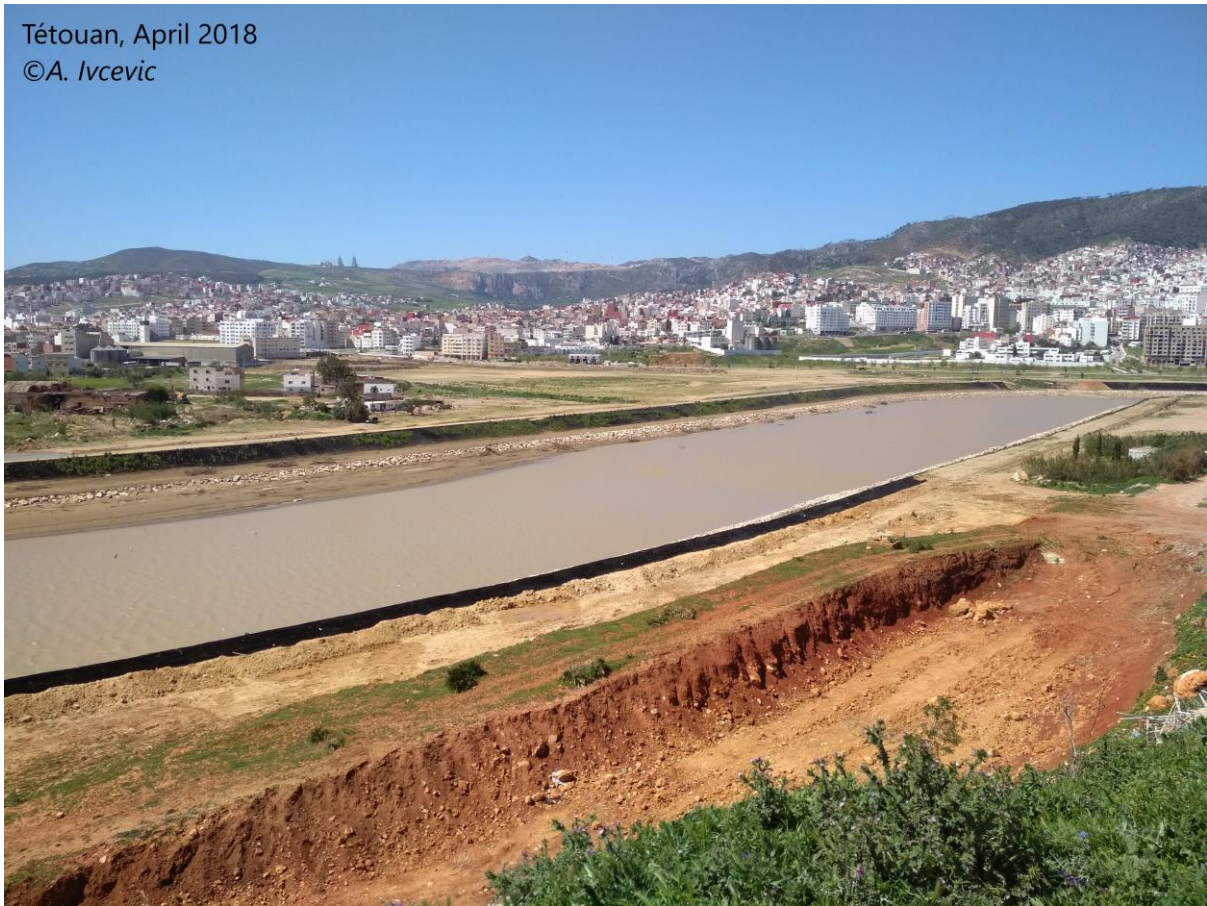
Figure 8: Construction site of Martil River floodplain in Tetouan.
