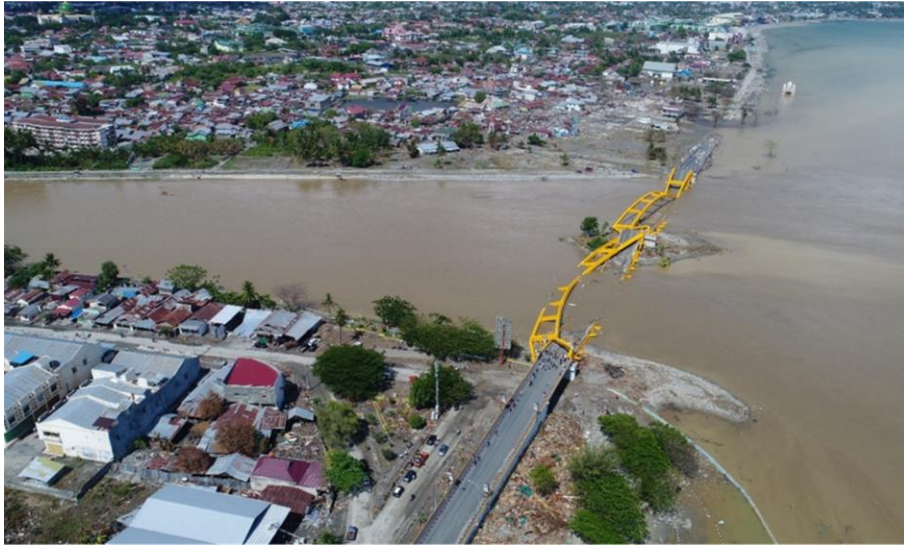
Figure 1: Palu, Indonesia, after a 7.5 Magnitude earthquake on 28 September 2018 (Syamsidik et al., 2019)
