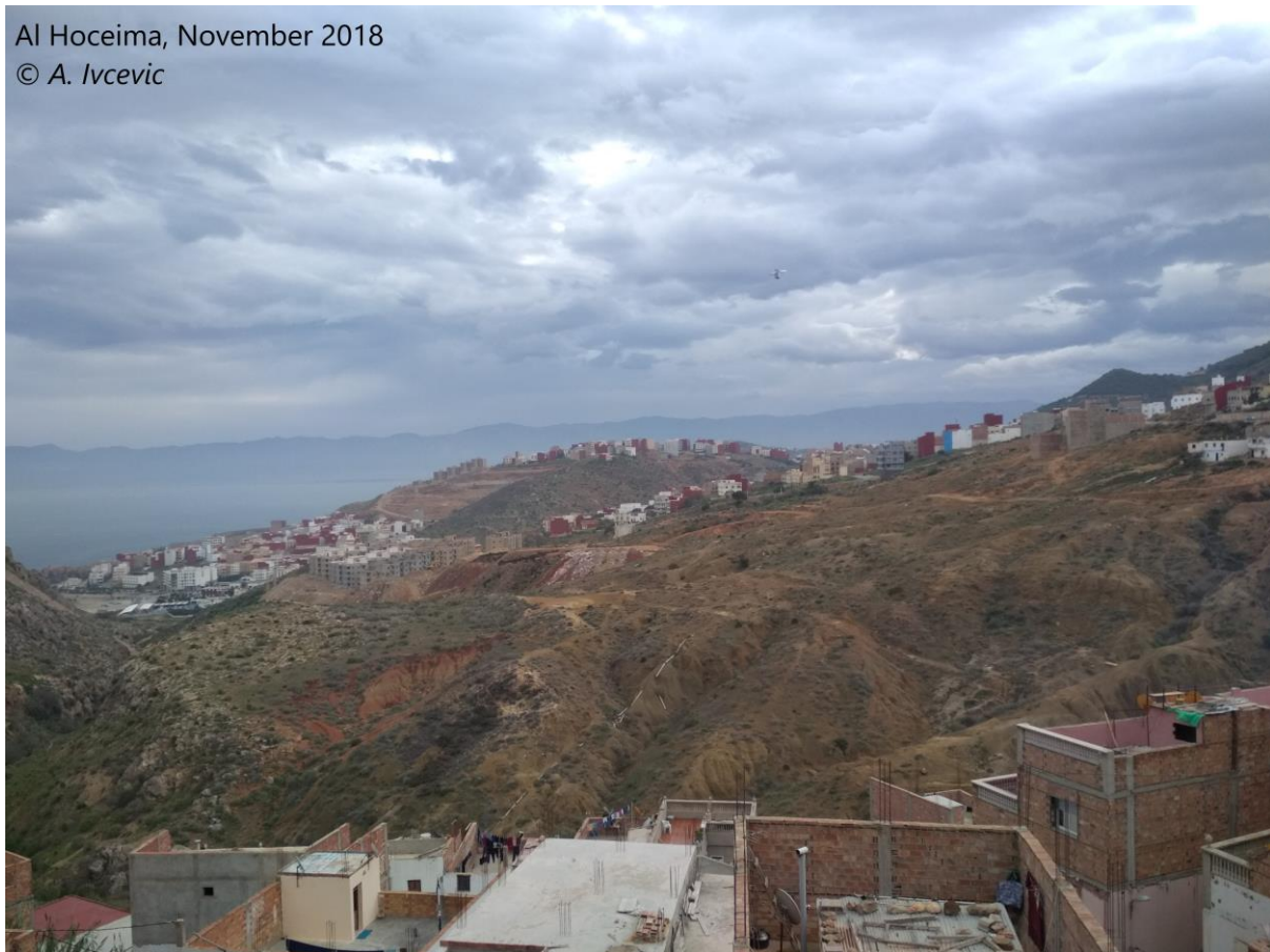
Figure 9: The construction sites in Al Hoceima, exposed to landslides, flash floods and seismic risk.
