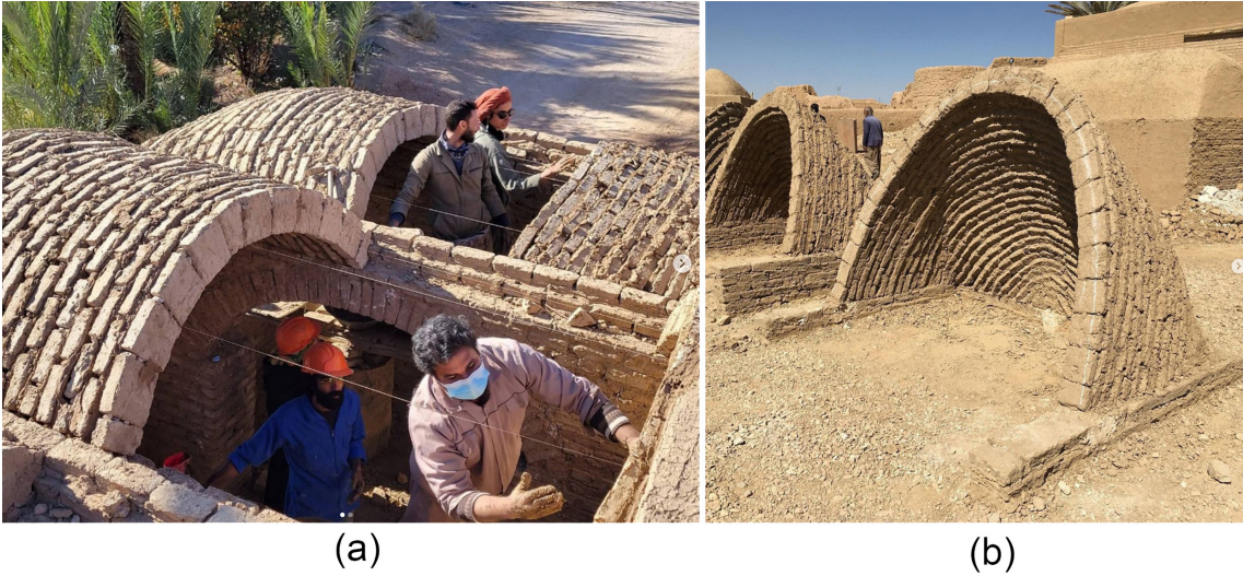
Figure 1.5 – Ground-Supported Barrel Vault
