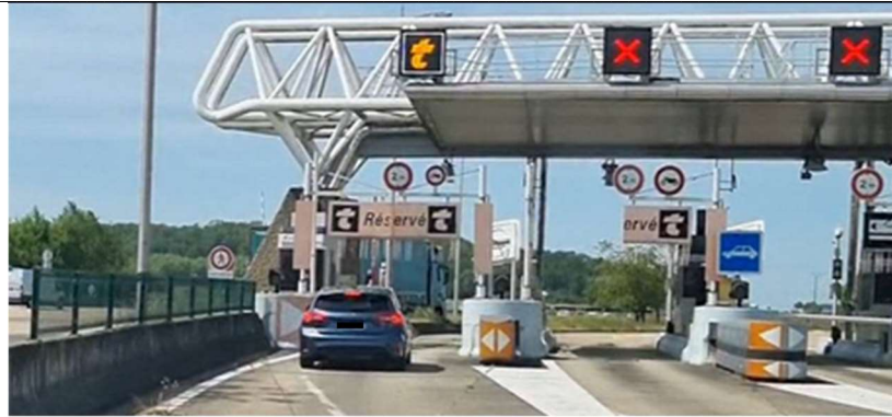
Figure 5.2. Open lane for testing
