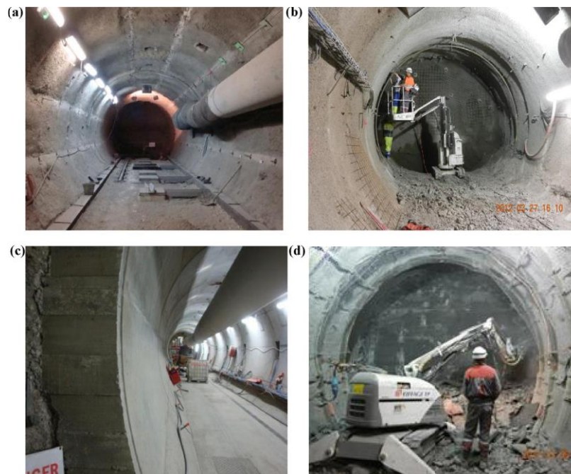
Figure 2.15. Excavation and support of galleries (Armand et al., 2013): (a) GCS with compressible concrete wedge, (b) GCR with concrete lining grouted in place, (c) BPE with 0.45 m of shotcrete projected in four layers, (d) GED gallery with classical support, shotcrete and sliding steel arches.
