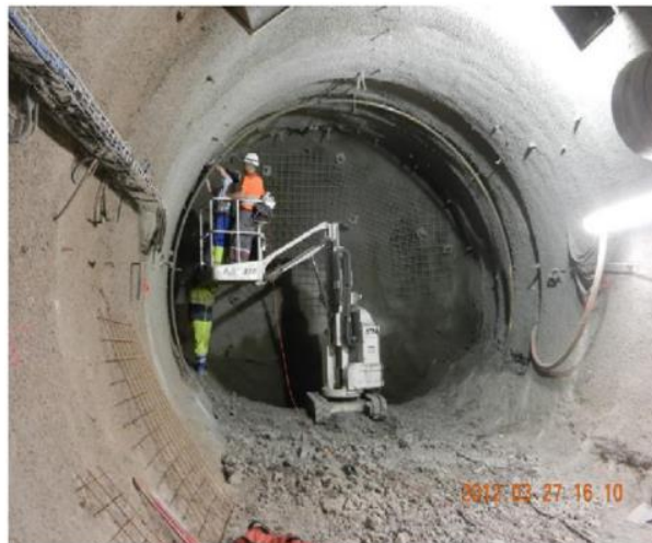
Figure 1.12. Gallery excavation (Armand et al., 2017)
