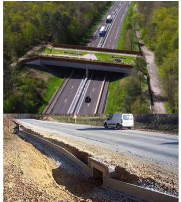
Fig. 2: Example of wildlife crossing structures: the Varennes overpass on highway A89, Puy-de-Dôme, France (top) and an amphibian underpass on road D14 (bottom, located in Doubs, France).
