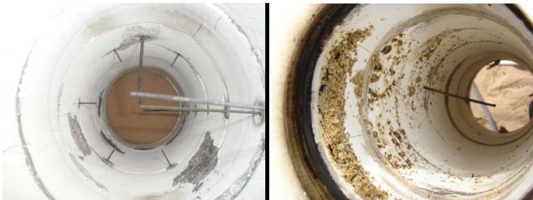
Figure (IV-17) - Photography of the reactor wall, after passage of the front.
