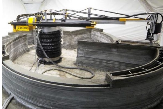
Figure 2.7: Apis Cor 3D printer machine.
