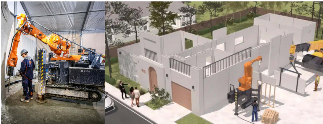
Figure 2.6: CyBe mobile 3D printer.
