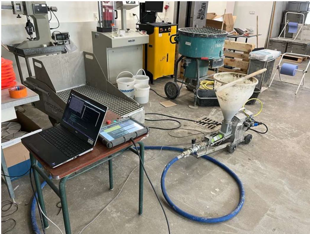
Figure B.8: Equipment installed in-situ, 27 September, 2023.
