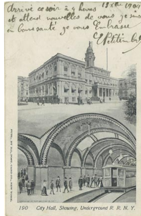
1904 City Hall, Showing, Under- ground R. R. N. Y.
