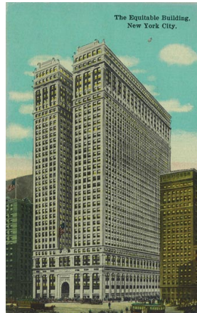
15 1913 The Equitable Building
