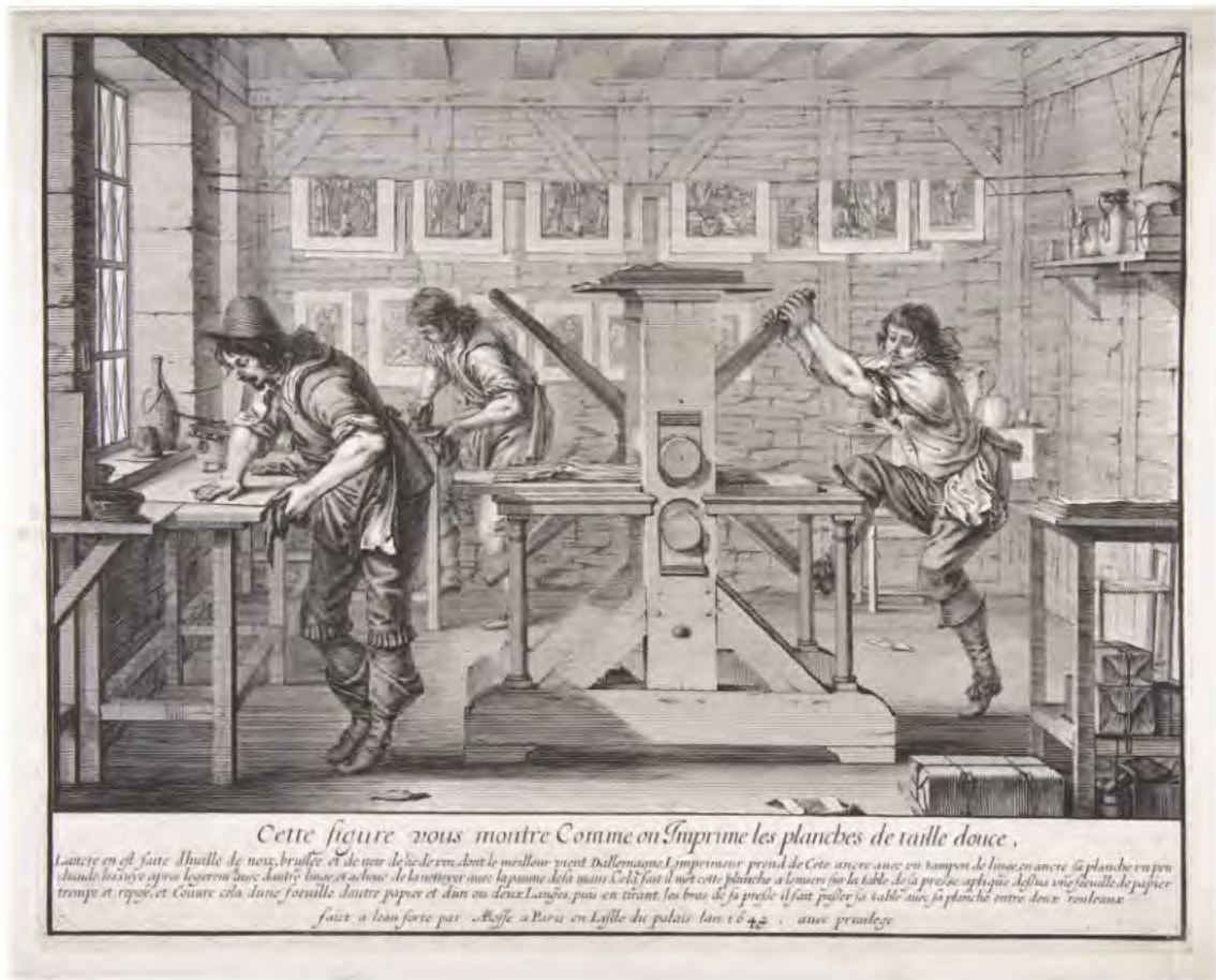
Fig. 5.10. “This figure shows you How Copperplates Are Printed.” The printing of copperplates differed substantially from that of woodcuts and movable types. In the latter, the figures appear in relief and the ink is applied to the raised surface. In the former, however, the figures are carved into the metal plate: the resulting grooves receive the ink, the remains of which are wiped off the surface. Unlike woodcuts and movable types, therefore, the printing of copperplates required much higher pressure in order to pull the ink out of the grooves. A special press was used, known as the rolling press. (Bibliothèque nationale de France, Paris.)
