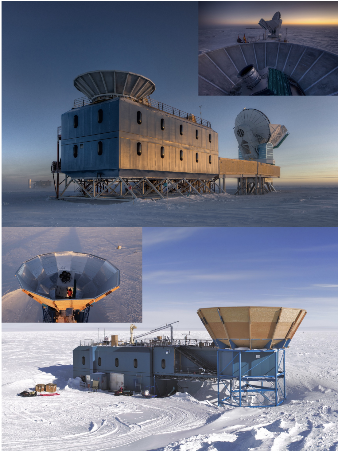
Figure 2.12: Top: a picture of the DSL, where we see the BICEP ground shield and the SPT, with a zoomed top view of the BICEP2 telescope, photos from Steffen Richter. Bottom: A picture of the MAPO from Willmert 2019, where we see the Keck Array ground shield, as well as a top view on the telescope. Picture from Robert Schwarz.
