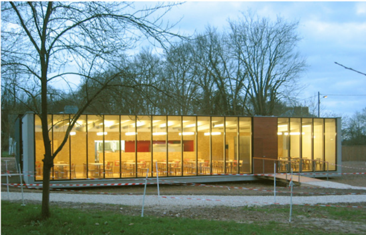
Fig. 35: After the construction of the central kitchen and restaurant of the Centre Saint-Martin, the director wished to change the modus operandi and include the members of the community in the development of a spatial transformation project (P. Marguc in co-contract with Drôles de Trames, 2006).
