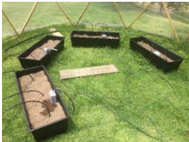
Figure V.3: Multiple sensors installed for data collection (4 soil moisture sensors, (1 air indoor sensor, and 1 weather station)
