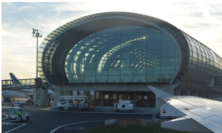
(a) CDG Airport Terminal 2E: Basket-handle profile shell with W^{2,\infty} -regularity
