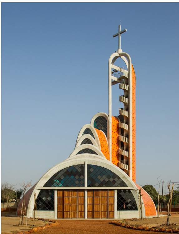
Figure 4: Nianing Church, Senegal. The project draws inspiration from termite mounds for passive thermal regulation (Regis L’Hostis/IN SITU ARCHITECTURE).
