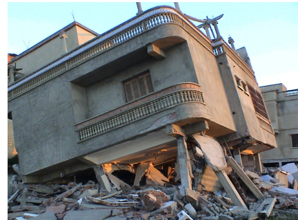
Figure 1.1: Effect of the soil-structure interaction (Ele, 2017)
