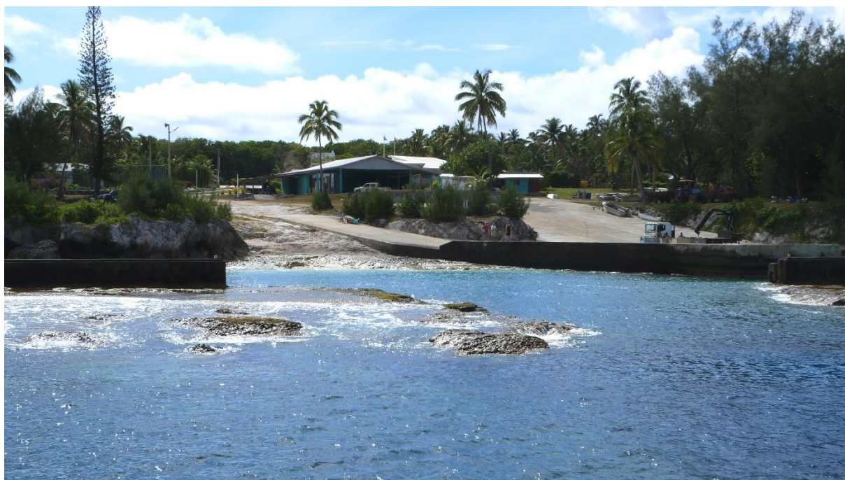
Figure 10 - Installation portuaire de Ma'uke (photo D. Glory, 2016)
