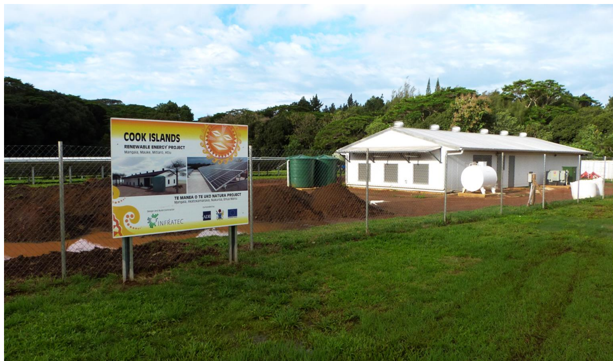
Figure 11 - Station solaire de Ma'uke (photo D. Glory, 2018)
