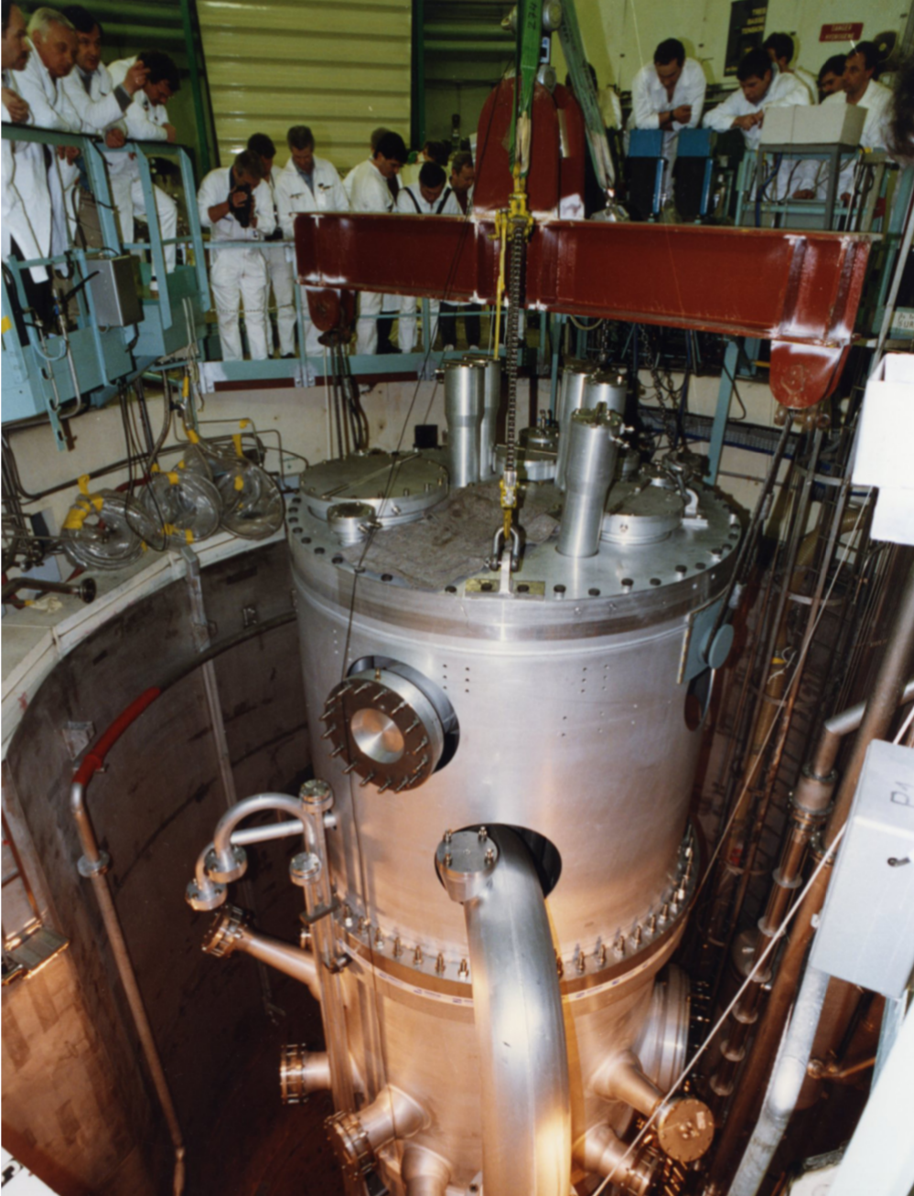
Figure 2.8: Installation of the reactor vessel in the light water pool [JAC06]
