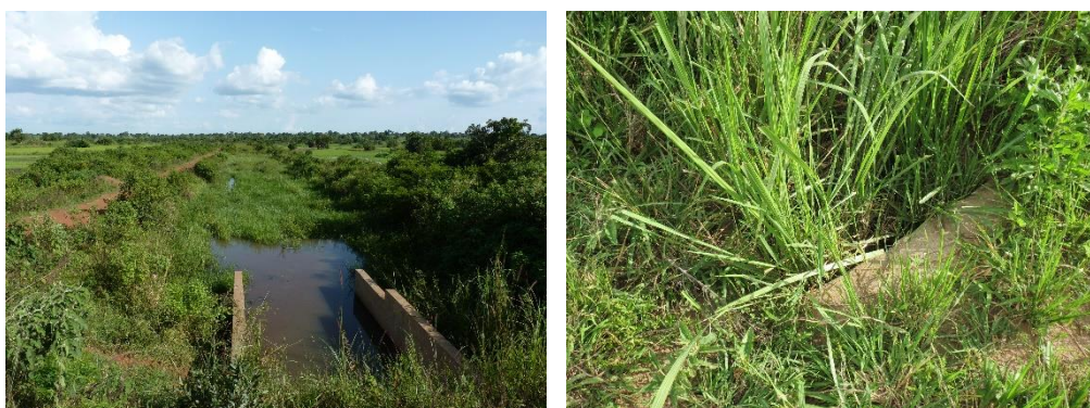
Picture 9 (left): View from the main dam of the main drain in Itek filled with silt and vegetation in the rainy season (Torretti 2014)
