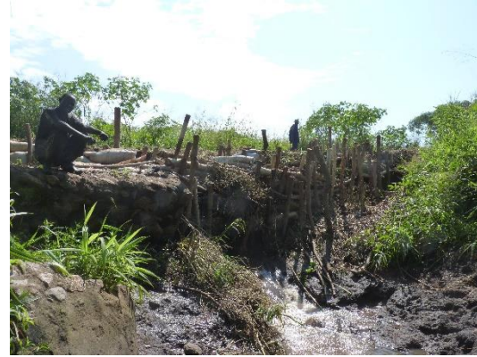
Pictures 23 & 24: WUA members diverting water through a page early in the rainy season (Torretti 2016)
