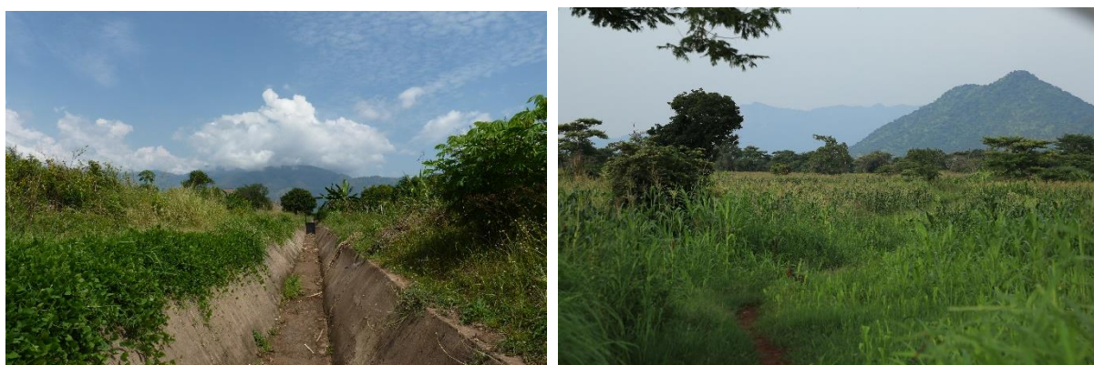
Picture 35 (left): Abandoned cemented canal in the northwest of the scheme in the rainy season (Torretti 2016)
