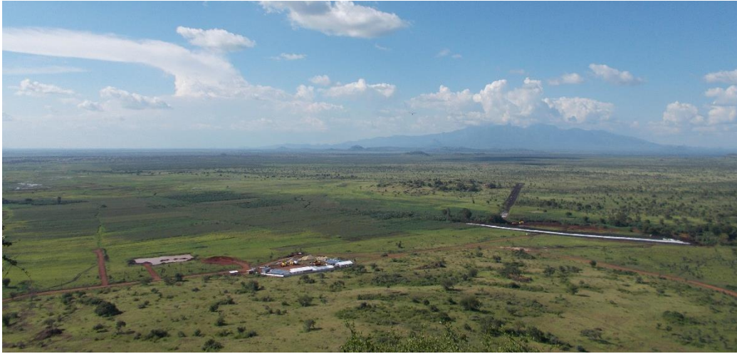
Picture 54: View of the Ngenge irrigation scheme under construction (Auffray 2018)
