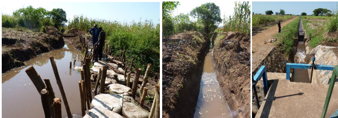
Picture 44 (left): WUA's page diverting the Okura stream through a hand-dug canal (background) in the rainy season (Torretti 2016)
