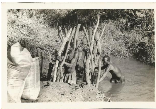
Picture 21 (left): Construction of an indigenous page for the irrigation scheme (Ocen K. 1969)
