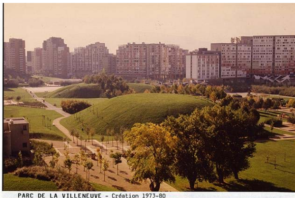
Figure 3.72 Jean-Verlhac Park at the end of the 1970s (Photo ©AMMG) 119
