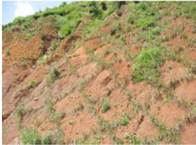
Photo 114: Applications of Vetiver grass for landscape stabilization (GTZ-IFSP/ South Gonder,2005)
