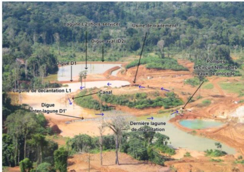
Mining dam system in a primary gold exploitation in FG (MSMg-type) showing a closed-circuit functioning. D2 is the most downstream dam (Barras, 2010)
