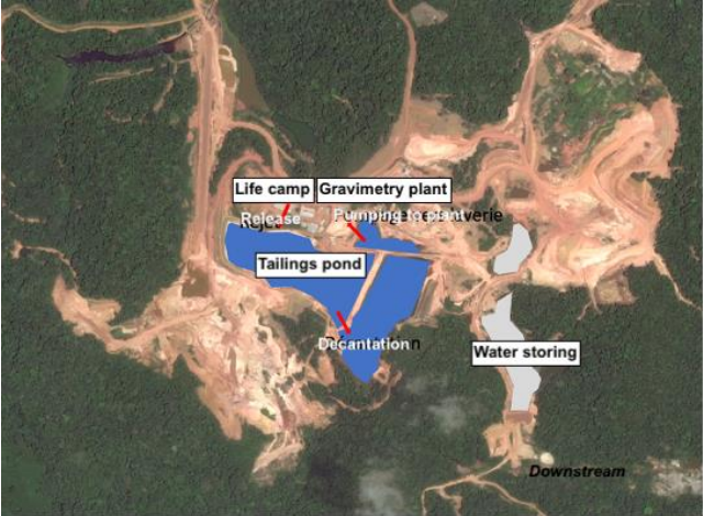
Figure 49 Simplified scheme of the tailings and water ponds in a MSMg-type in FG based on a satellite image. Source: Modified from Google Map, 2020 Maxar Technologies
