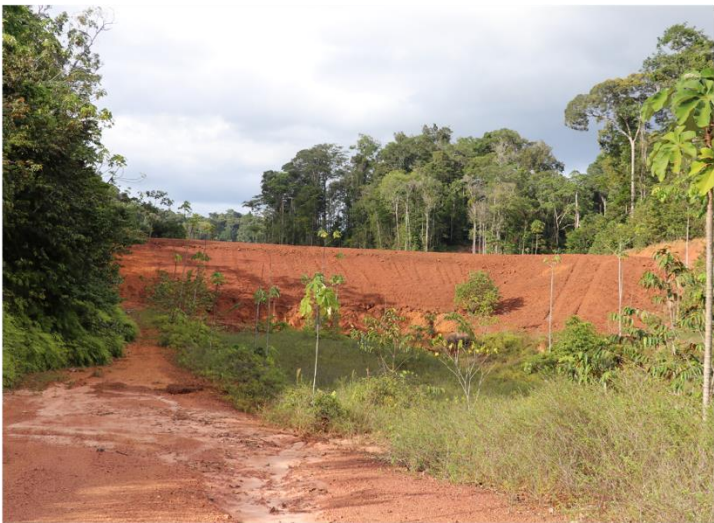
Figure 50 A mining dam in a MSM-type in FG
