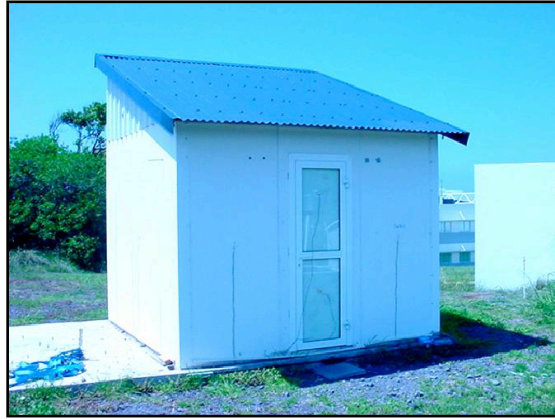
FIGURE 1. CELLULE LGI (IUT SAINT-PIERRE)
