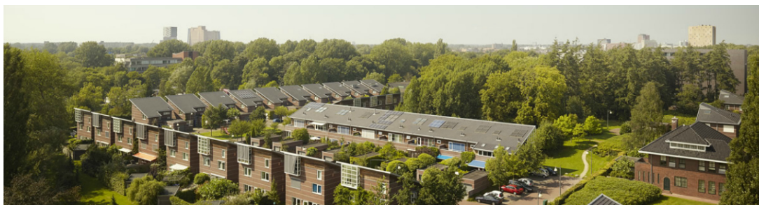
Figure 1.5: A smart-district in the Hoogkerk village, the Netherlands [44].
