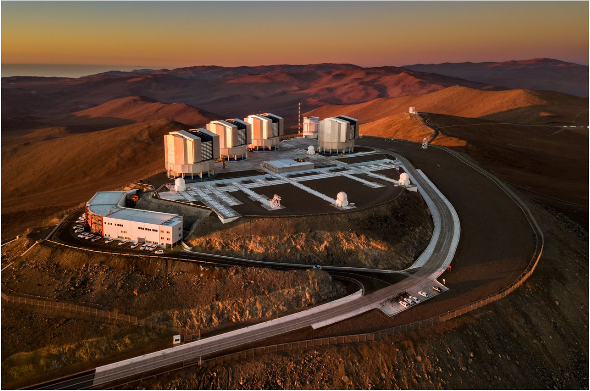
Figure 3.11 – Aerial view of the Very Large Telescope’s observing platform, installed at the Cerro Paranal Observatory (Atacama desert, Chile). The 4 fixed 8-m telescopes and the 4 movable 1.8-m telescopes are shown here. Source: https://www.eso.org/ .
