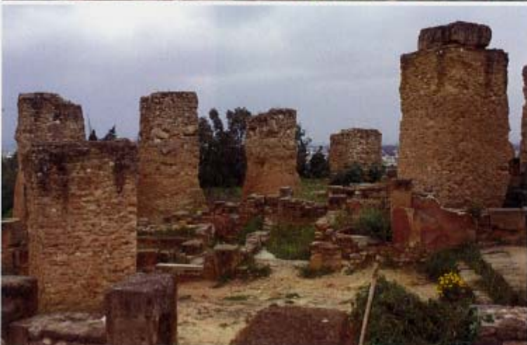
c: Detailed view of the columns in "pise" erected by the Roman, when, some years after the destruction of Carthage, they have refilled the slopes of the hill of Byrsa for levelling a new platform which will bear the new Forum and Basilica of the Roman Carthage (1 st Century A.D.). This structural performance consisting in building earthen columns for realising new footings is in fact common in the Roman engineering practices. Other similar traditions are existing in the history as this can be observed at Susa, Khuzistan, on the Darius' Palace.
