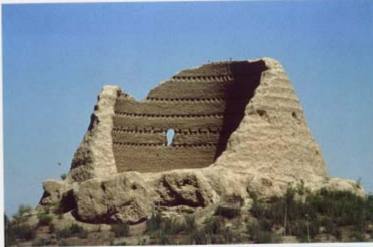
a: On the same site of Ancient Merv, visitors can observe an impressive structure built in unbaked earthen bricks; a ice house. This tradition of such big structures used for storing the snow, the ice and the cold water in big tanks deeply embedded in the ground is one of the permanent feature of the vernacular architecture of the Central Asian region.
