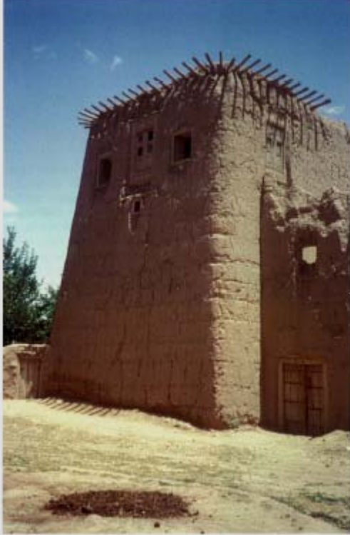
a: In Afghanistan, close to the border of Pakistan, an example of local typical fortified rural houses, or farms, build in "cob". This building culture, in numerous regions of Afghanistan, is much more present than the adobe construction and locally called "parsha".
