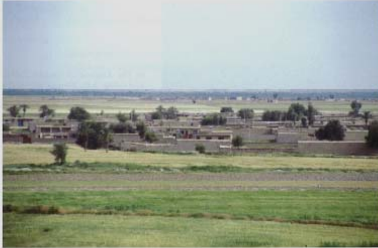
a: Typical feature of the traditional people's housing in earth valorising the technology of the "cob" (thick walls in stacked packs of mud) on the Plateau of Khuzestan. Here, the roofs are terraced and particularly adapted to a dry climate.
