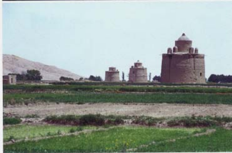
c: Still impressive is the famous tradition of the pigeons towers built in adobe and burnt bricks on the plateau of Isfahan, Iran. Here, by a locality called Gavart (between Isfahan and the airport), and all around, most of the traditional villages are mainly built in " khesht " (unbaked brick), plastered in " kha-ge! " and exhibit the blooming of the Persian traditional know-how that have produced an earthen architecture in vaults and cupolas.
