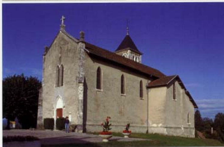
c: A rare and nice example of a Christian church built in "pisé", plastered with a thin lime distemper, in Isere, village of Charancieu located around 30 km north Grenoble. This church has been built at the middle of the XIX e Century. All walls, excepted those of the bell tower are in "pisé".
