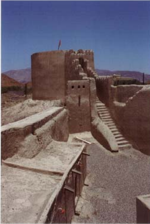
a: The Sultanate of Oman testifies of a very nice earthen architecture built in unbaked earthen bricks which have been traditionally conical-shaped and recently evolving to the common rectangular shape. This traditional earthen architecture of the Sultanate covers numerous examples of Forts with massive outer defensive walls and towers, or "bors", and a nice tradition of outdoor and indoor plastering in "suroof" (natural lime) or "jusi" (gypsum) as well as earth and straw. Here the Fort of Bid Bid, on the road from Muscat to Nizwa. The Fort of Bid Bid has been restored during the 80's of the last XX e Century by the Ministry of National Heritage of Culture which has recently conducted new restoration works valorising the aesthetic of the traditional renderings.
