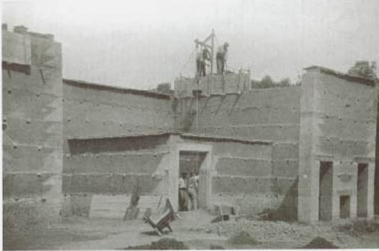
a: This photograph taken at the beginning of the XX e Century, circa 1914-20, is showing the common practice of the "pisé" construction (rammed earth) in the Province of Dauphiné, region of Isere, northern of Grenoble (South-East of France). At that time, a typical evolution was introduced in the practice of "pisé" with the use of the concrete, replacing the traditional corner-stone, the quoins in burnt brick-work or in lime mortar, or for consolidating the reveals of the bays.
