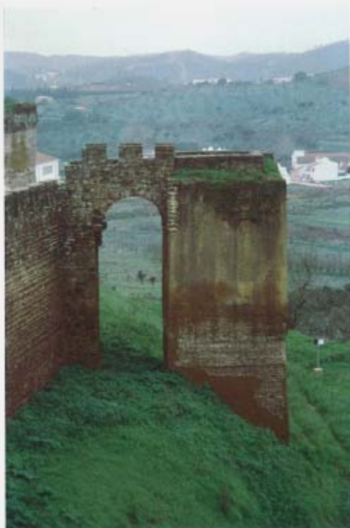
a: The remains of the Castle of Silves, Province of Algarve, South of Portugal. The tradition of fortified castles tracing back to the period of "Al-Andalus" (Moore times) testifying of the construction in "pise" ("taipa") is quite common in this region of Portugal where several projects of conservation have been launched.
