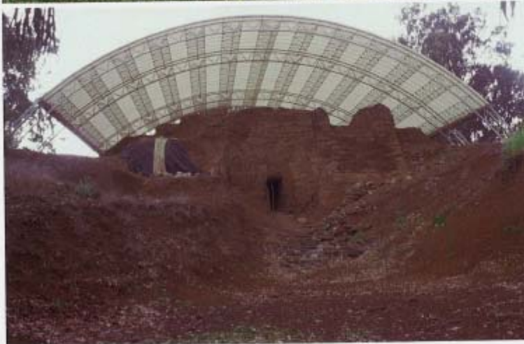
c: View of the eastern façade of XVIII th Century B.C. (Middle Bronze Age) gate of the Canaanite city of Laish at Tel Dan, northern Israel. This famous triple arched gate in unbaked bricks of Tel Dan (built in three radial courses) the span of which is about 2.50 m, has been excavated by Professor, archaeologist, Avraham Biran. It is part of a defence system which consisted of sloping ramparts and glacis. Stone constructions have been found, built against and close to the mud structures whose successive layers are made with brown and grey coloured bricks.
