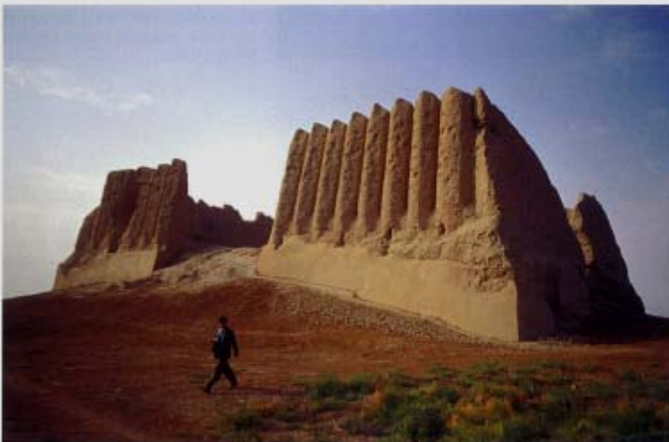
b: In Turkmenistan, the famous medieval site of Ancient Merv which has been entered on the List of the World Heritage of UNESCO in 1998. The original architectural design of the outer walls of the "Great Kyz Kala", built in unbaked bricks during the XI th and the XII th Centuries A.D. is today known as a "corrugated" structure the shape of which having been compared with other structures of a similar type existing in Iraq.
