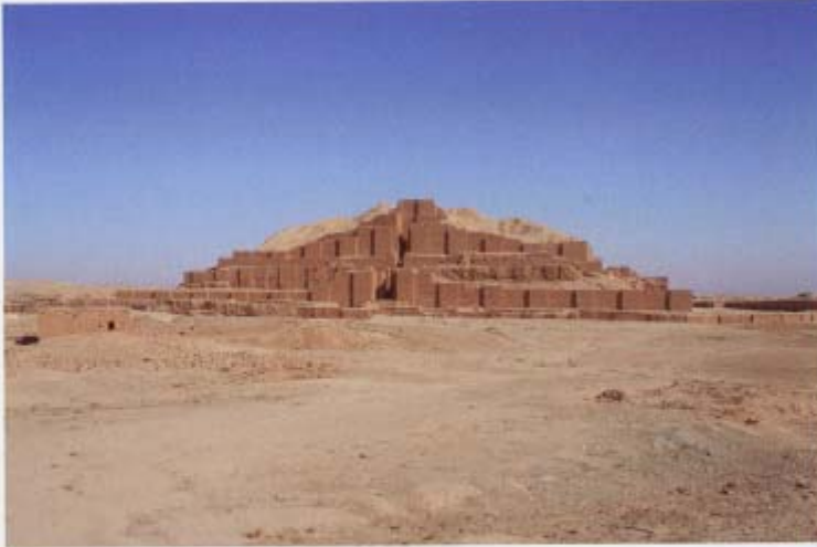
a: The Ziggurat of Chogha Zanbil, Khuzestan, Iran, Elamite site of the XII th Century B.C. On this site, the unbaked earthen brick or " Khesht " in Persian, still has been the main building material for the construction of the core of the structures, not only for the Ziggurat itself but also for other main significant structures as the temples located in the Temenos area or the Hypogeum palace and other royal palaces and massive gates. But on the Ziggurat, the structural components have been protected with burnt bricks while all plastering devices for the outside protection have been made in " kha-ge! " or clayey mortar amended with chops of straw.
