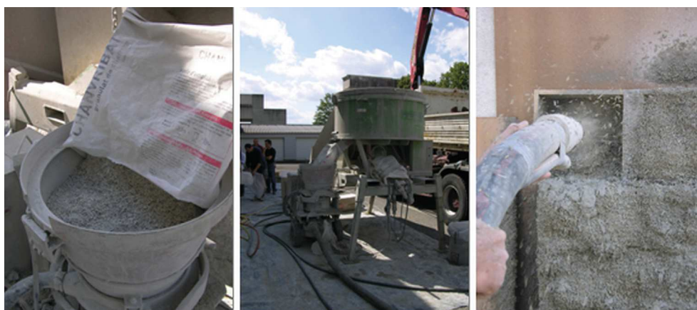
Fig. 5. Device for spraying hemp concrete (SHC) – dry mixer, shutter.
