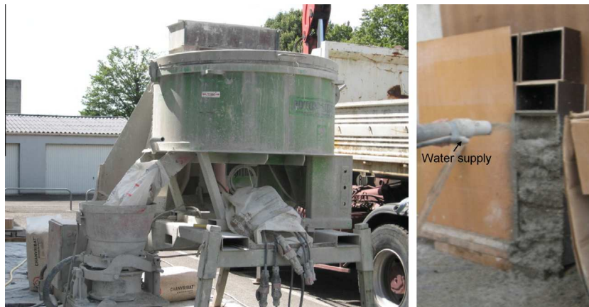
Fig. 1. Spraying method (left: mixer, right: spraying hose).
