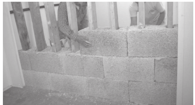
Fig. 4. Building of the test wall.
