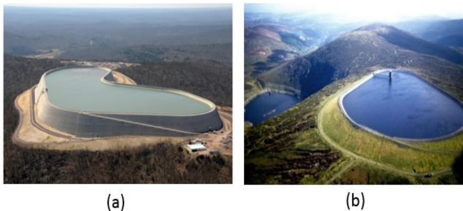
Fig. 31: Examples of upper reservoirs with a man-made reservoir wall (a): Taum Sauk PHES [199], USA (b): Turlough Hill PHES [200], Ireland.
