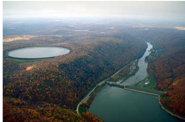
Fig. 28: Example of dammed stream used as lower reservoir in PHEs scheme in northwest Pennsylvania, US 5 .
