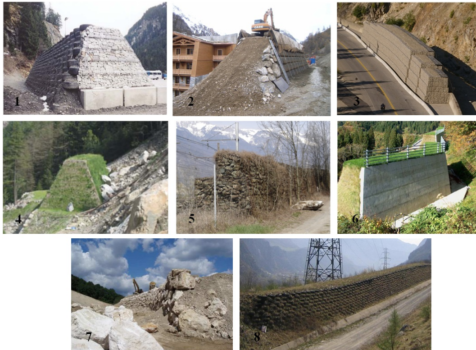
Figure 1.1 Various types of rockfall protection embankments, in terms of geometry, dimensions and constitutive materials. (for references, see Lambert and Bourrier [2013]).
