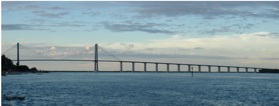
Figure 1.15: Rosario-Victoria motorway bridge, Argentina [Flores, 2007].
