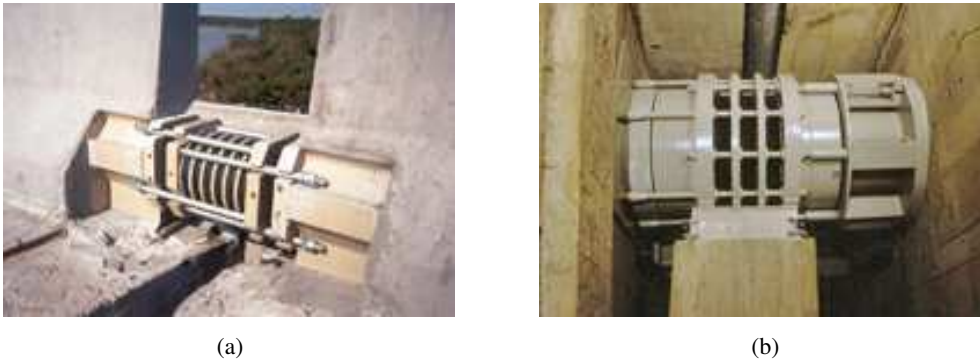
Figure 1.14: Elastic devices [FIP Industrial, 2016]: a) Devices installed along the "Conexion Rosario-Victoria", Argentina; b) devices installed in the Somplago flyover, Italy: the first seismically isolated European bridge (1974-1976).
