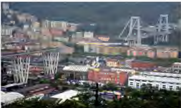
Morandi bridge collapse in Genoa (14/8/2018).
