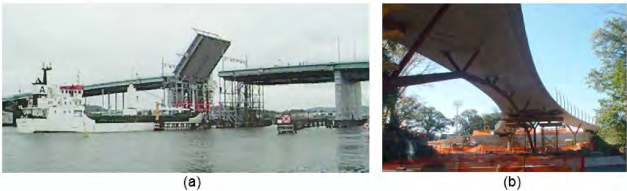
Figure 1-18: (a) Götaälv Bridge in Gothenburg, Sweden. (b) Streicker Bridge in Princeton, United States [47].
