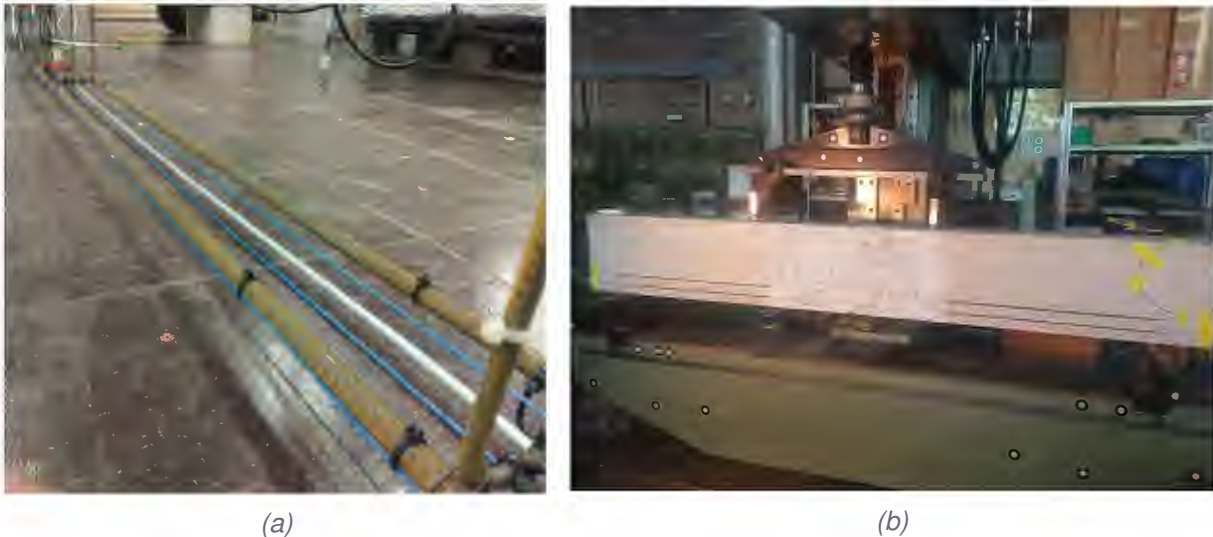
Figure 4-22: (a) Embedded optical fiber lines before concrete casting. (b) Front view of the loading arrangement and the textured area for DIC.
