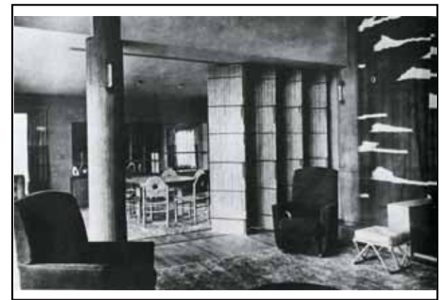
Living room and dining room, curtains drawn in front of the staircase on the right (1F)
