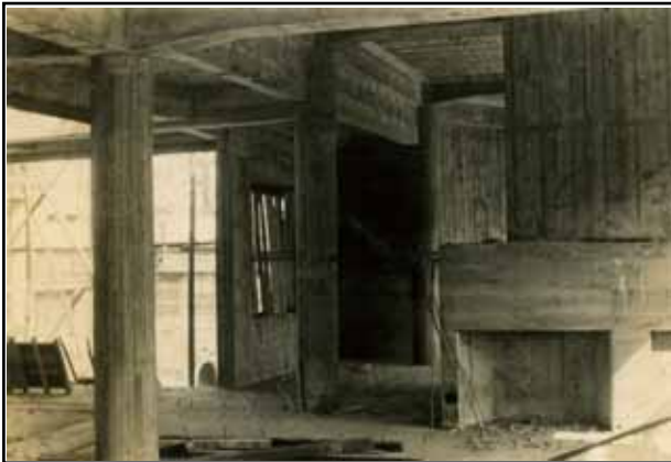
Building site: living room with fireplace on the right
