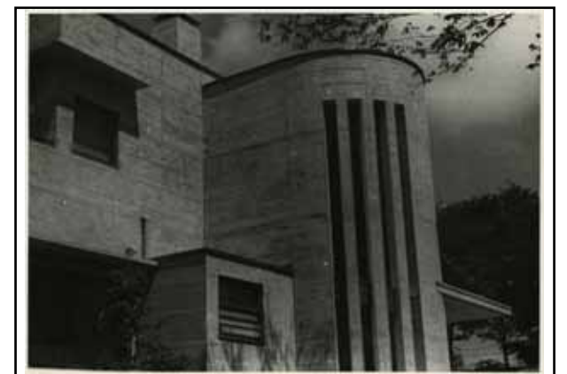
Staircase (east facade)
