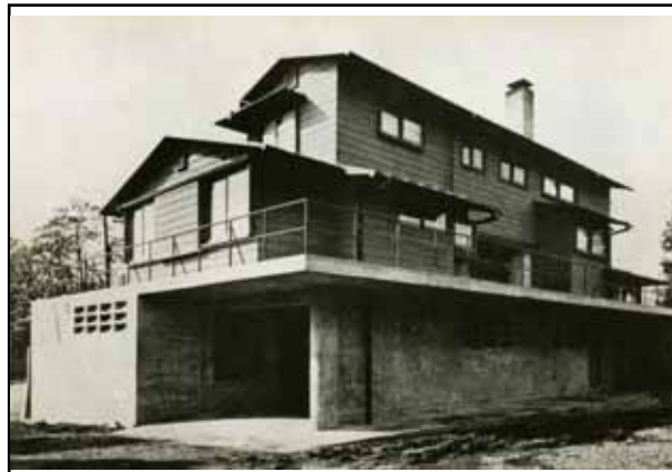
North-east view, with entrance to garage on east side
