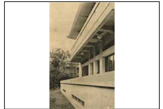
Terrace parapet (south)
