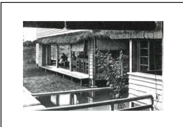
View of living room across from bedroom
