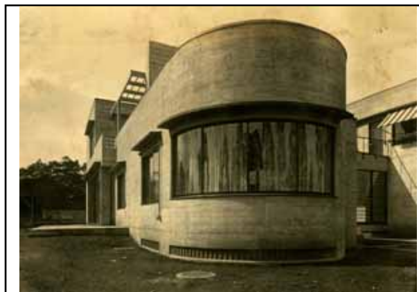
East facade (left part)
