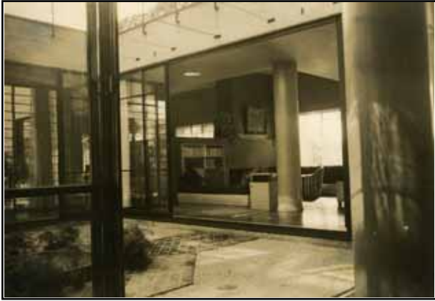
Patio with living room in the background
