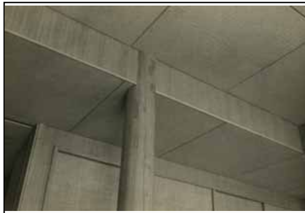
Ceiling and pillar (1F)
