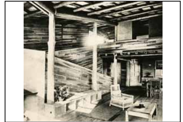
Living room with ramp and fireplace
