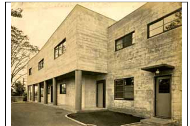
North facade (north-west view)
