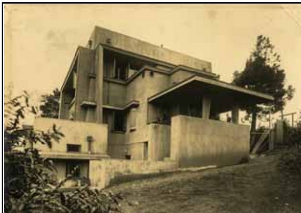
View towards entrance porch on the right (east)
