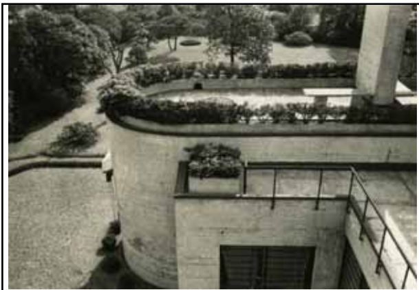
Roof garden above lounge
