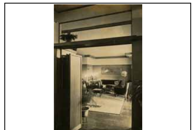
Living room seen from entrance hall (1F)
