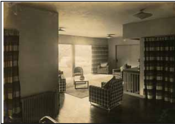
Sitting room with sliding doors opening onto Japanese room on the far right (1F)
