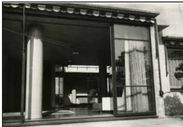
Living room sliding doors (south)
