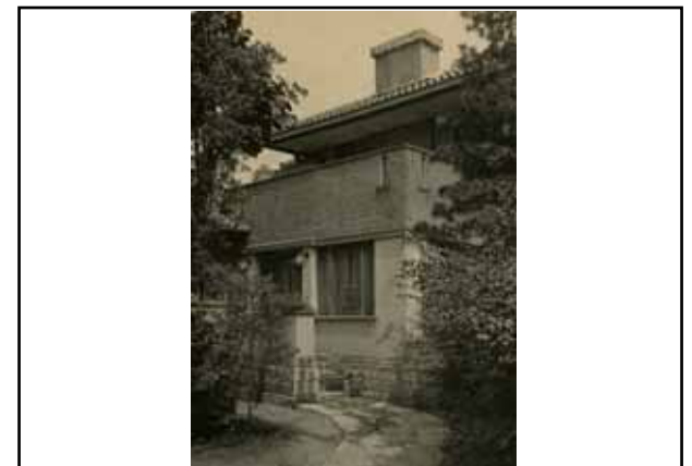
Stairs to service entrance (south-east)
