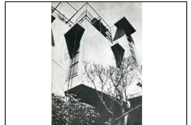
Second floor facade
