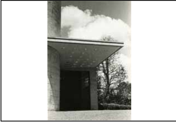
Entrance (east view)
