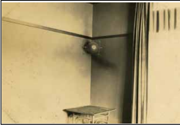
Room corner with light fixture
