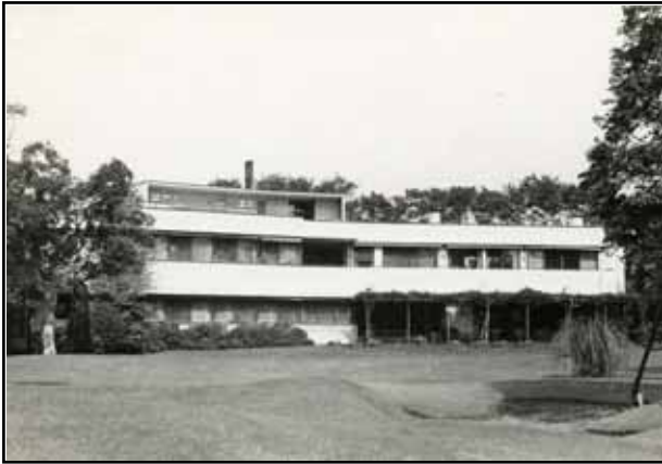
South facade with garden
