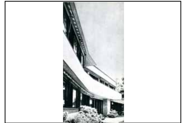
South facade (south-west view)
