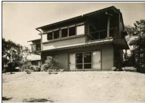
South facade with garden
