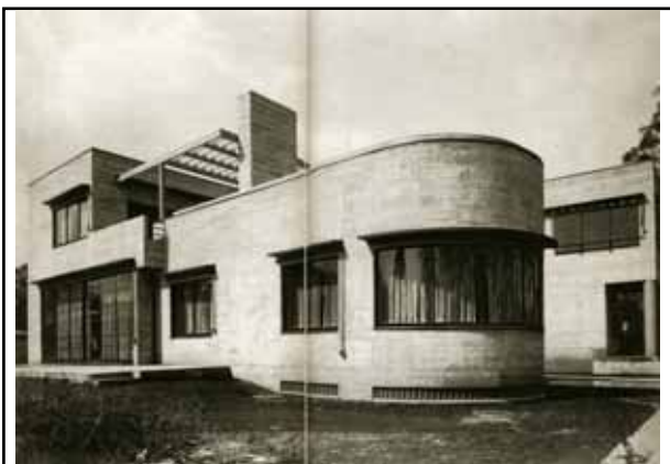
South facade (south-east view)
