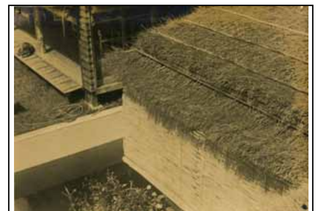
Thatched roof (larch)
