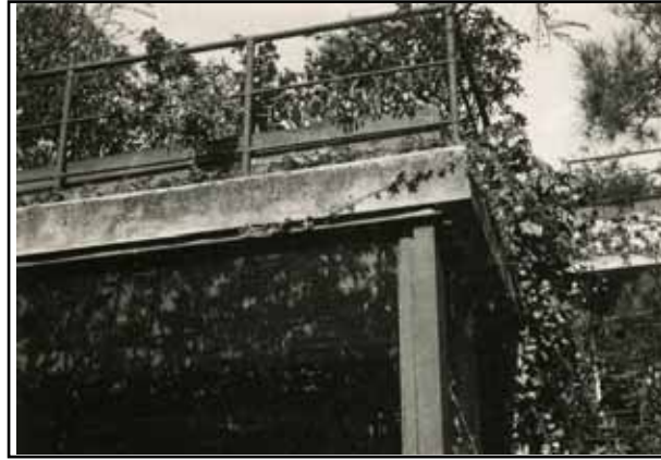
Roof garden handrail (on street side)
