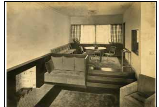
Living room and dining room in the background (1F)
