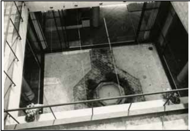
View of patio from roof garden
