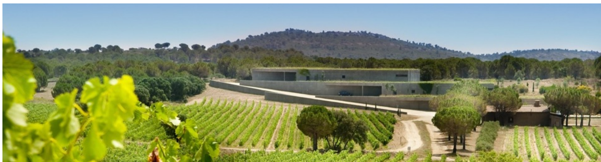
Photo 14 - Chai Terra Remota en Empordà - https://spanishwineexperience.es/
