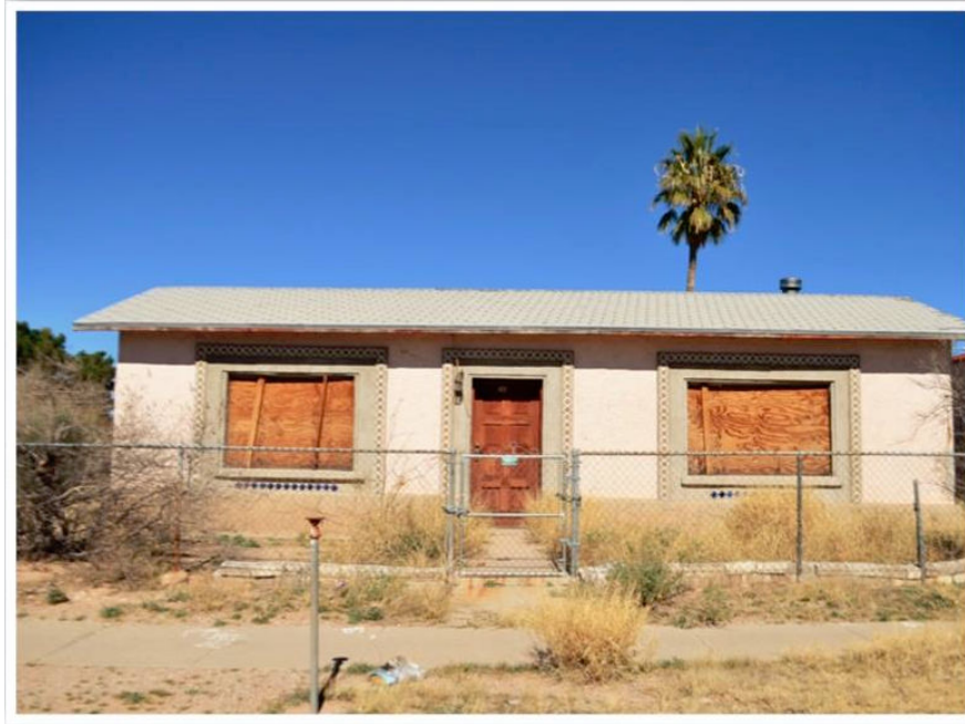
Picture 1: Stores in the South Side
