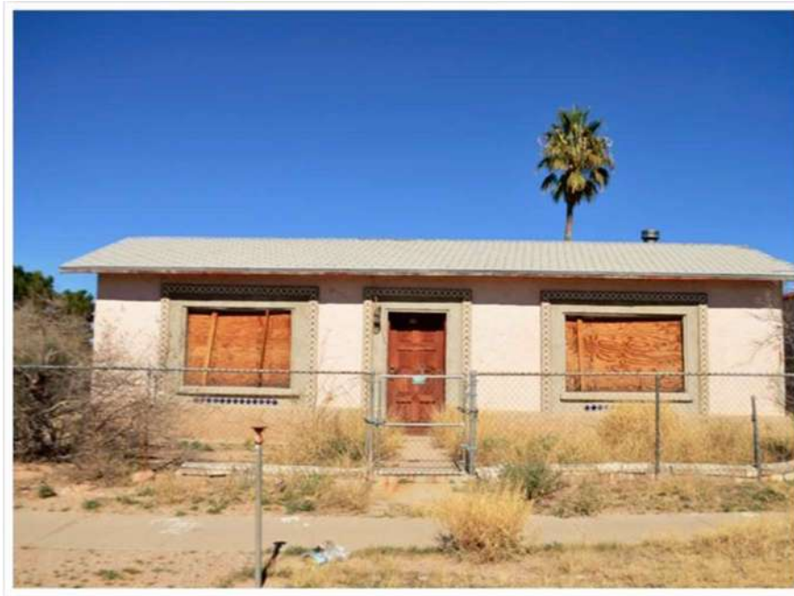
Picture 1: Stores in the South Side
