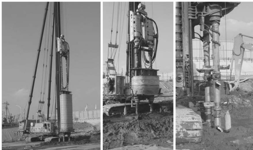
Figure 1-5 Equipment used for CDM (Topolnicki, 2004).
