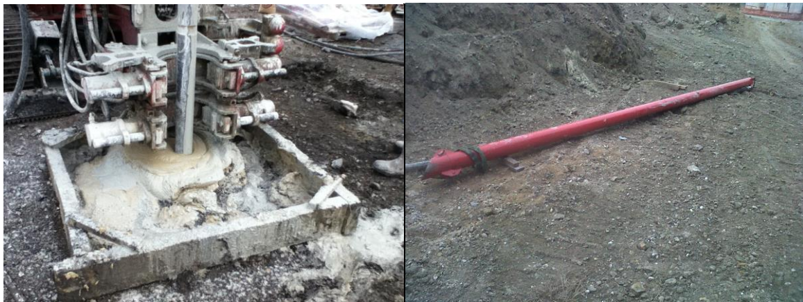
Figure 2-6 Spoil return to surface and sampling tube used for wet-grab samples.
