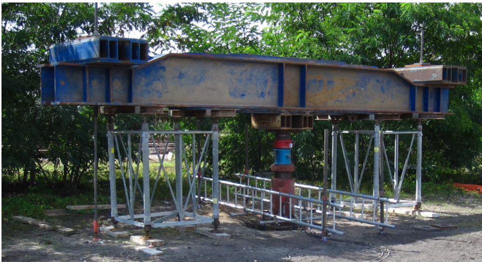
Figure 4-50 Set-up for static load test on column C2.
