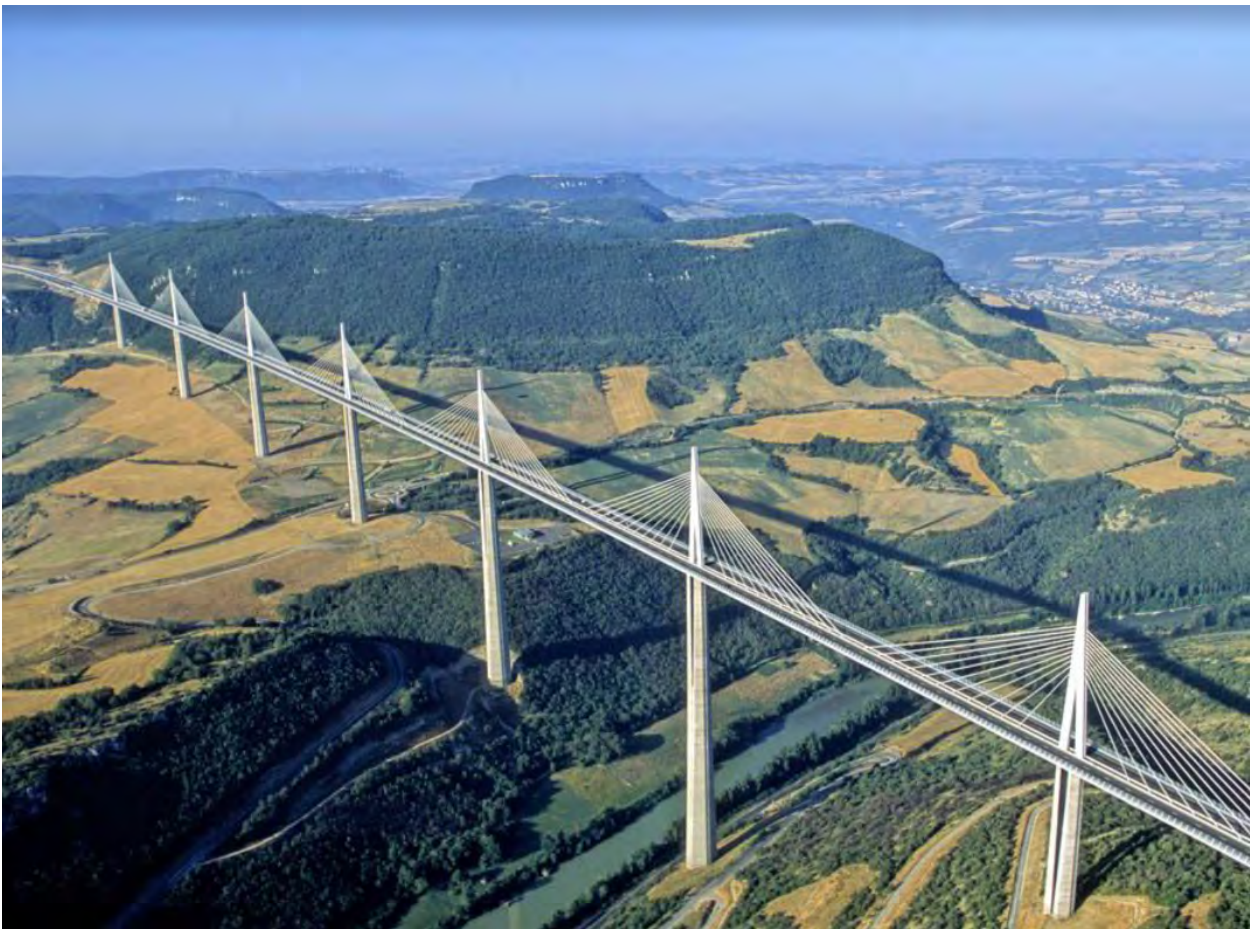
FIGURE 3.1 – Perspective view of the Millau Viaduct
