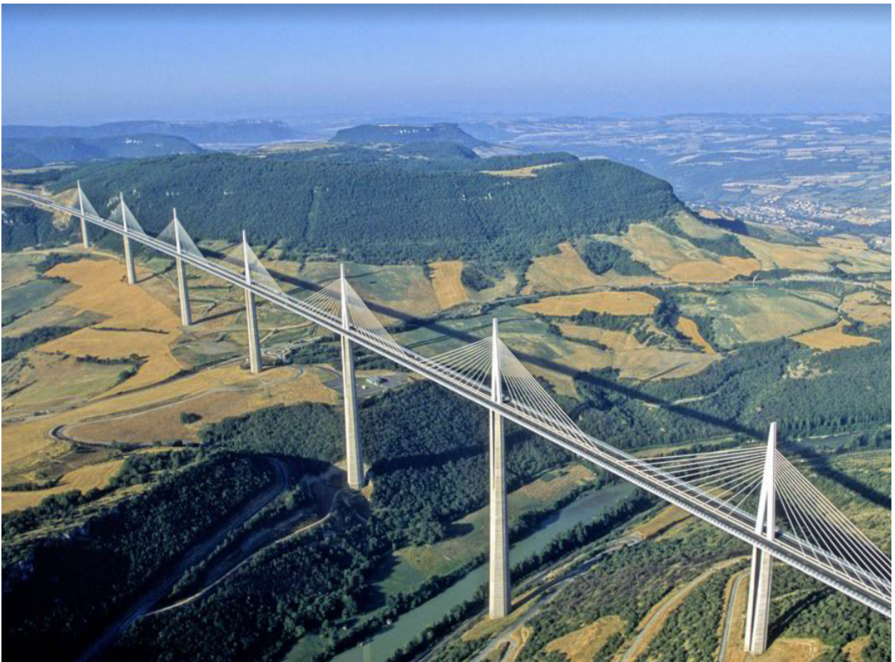
FIGURE 3.1 – Perspective view of the Millau Viaduct
